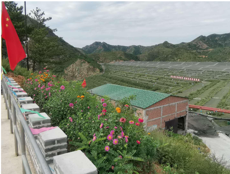
附属设施区砖砌挡墙
